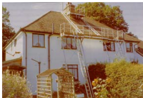
Figure 25 Proprietary access system for roof-work
