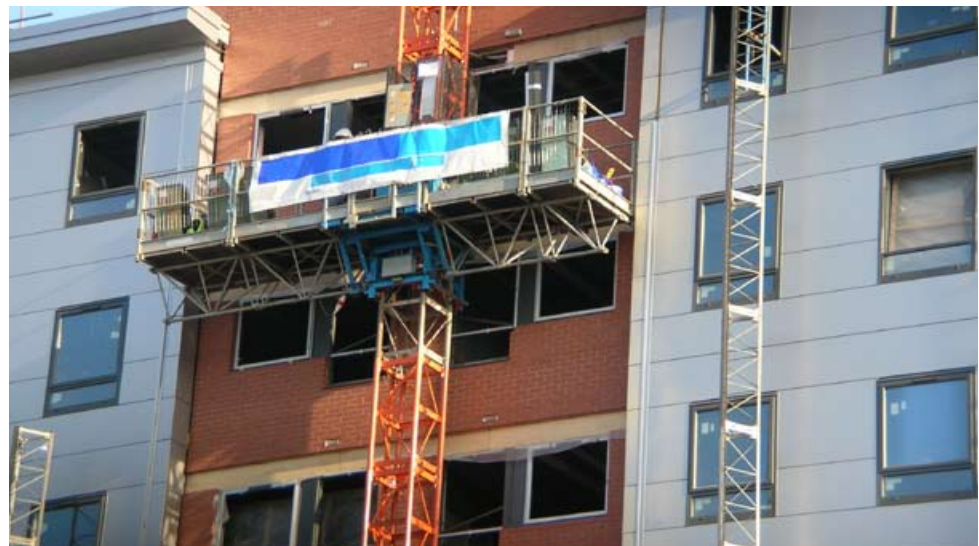
Figure 14 A mast climbing work platform
