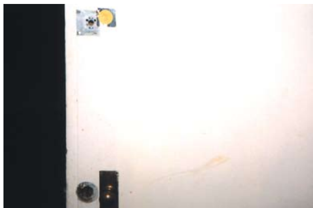
Figure 48c Painted asbestos insulating board facing to a fire door with some damage around the door furniture
