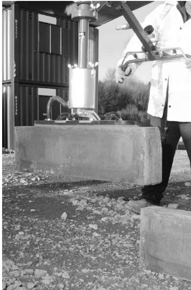
Figure 38 Handling kerbs using a vacuum lifter
