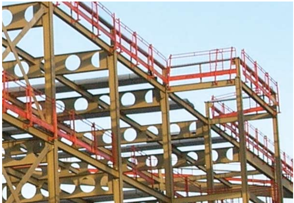
Figure 28 Edge protection installed with the steelwork
