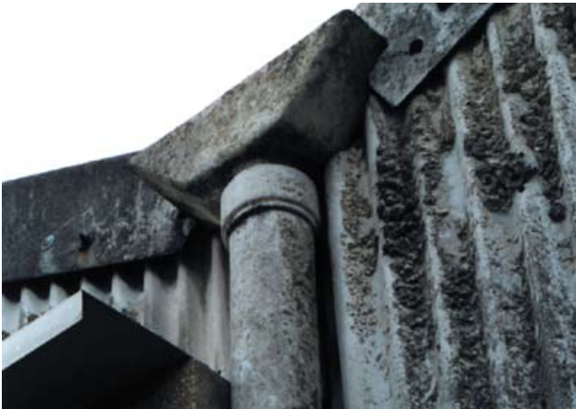
Figure 48d Asbestos cement downpipe, hopper and profile sheet
